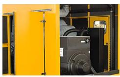
The front and rear sound attenuators can be removed to reach the alternator and radiator for scheduled maintenance.
