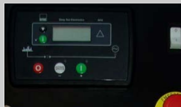
Deep Sea Controller with Panel Isolator and emergency stop
